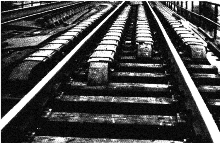
Fig. 23. View of the protection of the ends of the rail bundles from being hit by a protruding element in the event of faults in rolling stock (Miklin & Sawicki, 1993)
